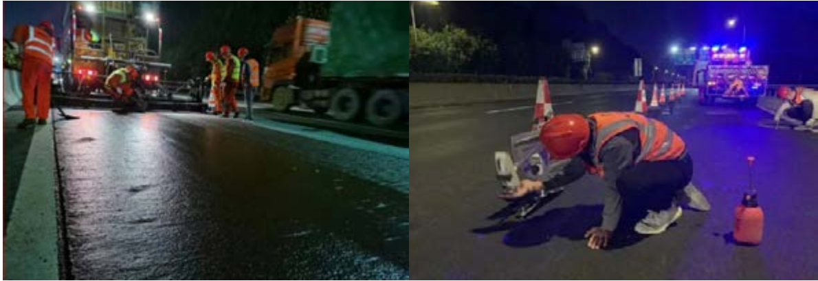
Emulsified asphalt with high viscosity and high elasticity is applied in pavement of North Second Ring Expressway
